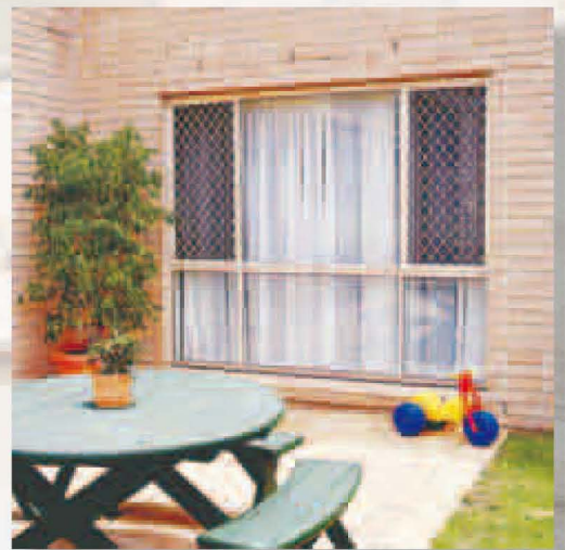
Window grilles to sliding sashes only
